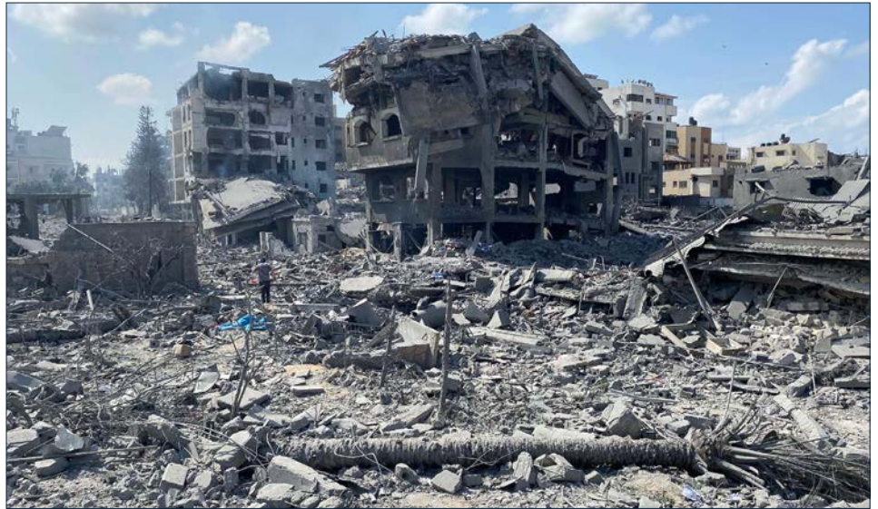
Damage in Gaza Strip during the October 2023.
