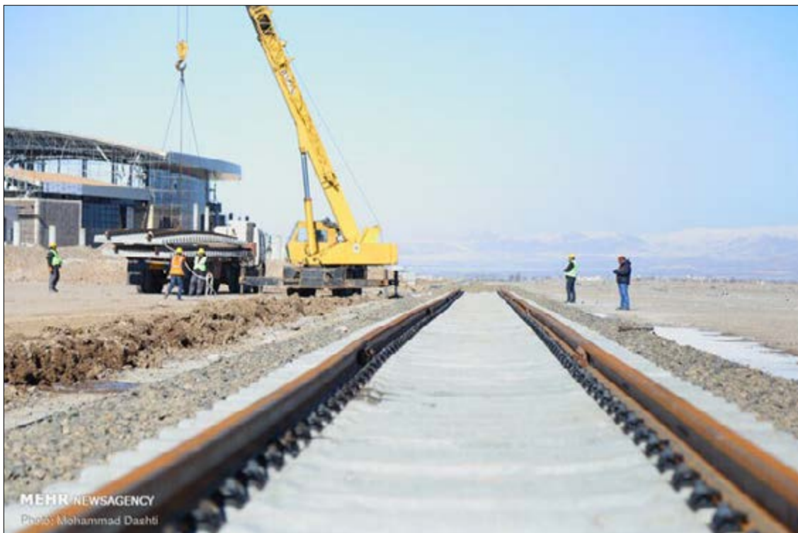
The Chahbahar-Zahedan railway under construction. Source: Mehr News Agency, https://media.mehrnews.com/d/2020/10/21/3/3585307.jpg
