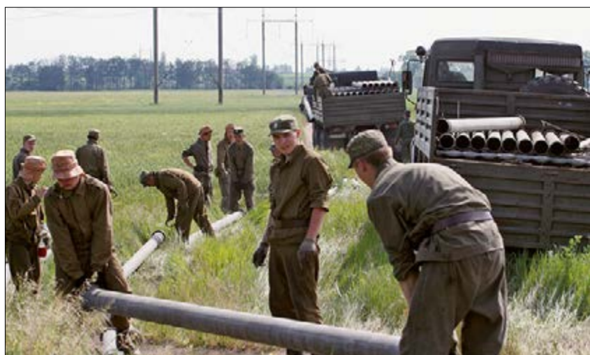
Russian military forces preparing to lay water pipe in Crimea, August 2020.
