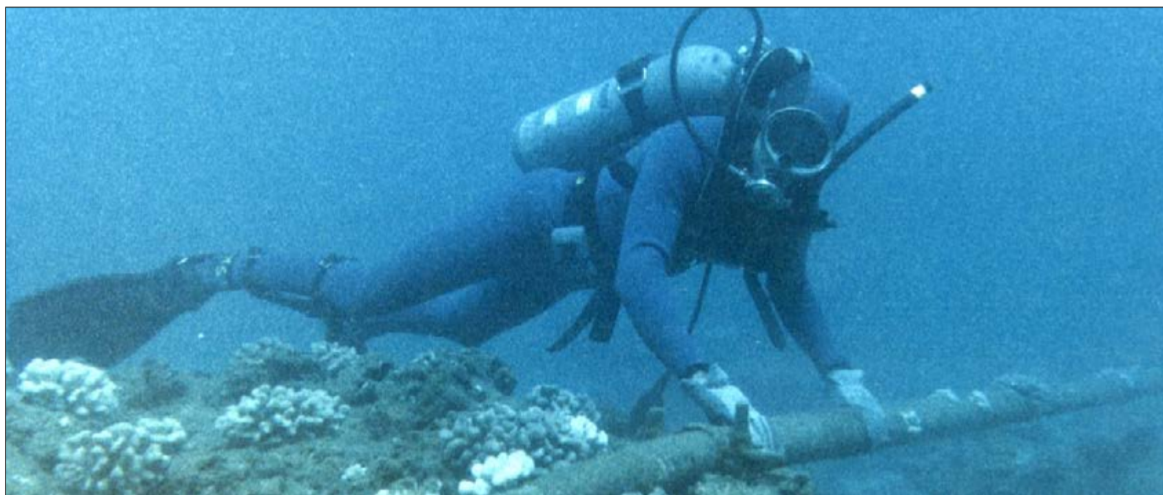
Diver Checking Underwater Cable.
